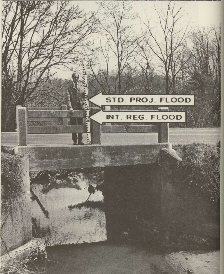
Hydraulic Road Bridge
