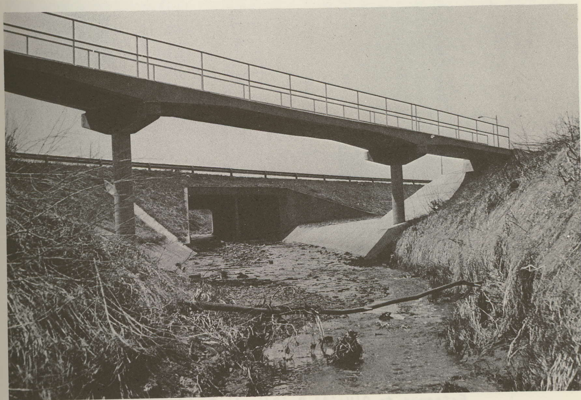
Pedestrian crosswalk and U.S. Route 250 Bypass
