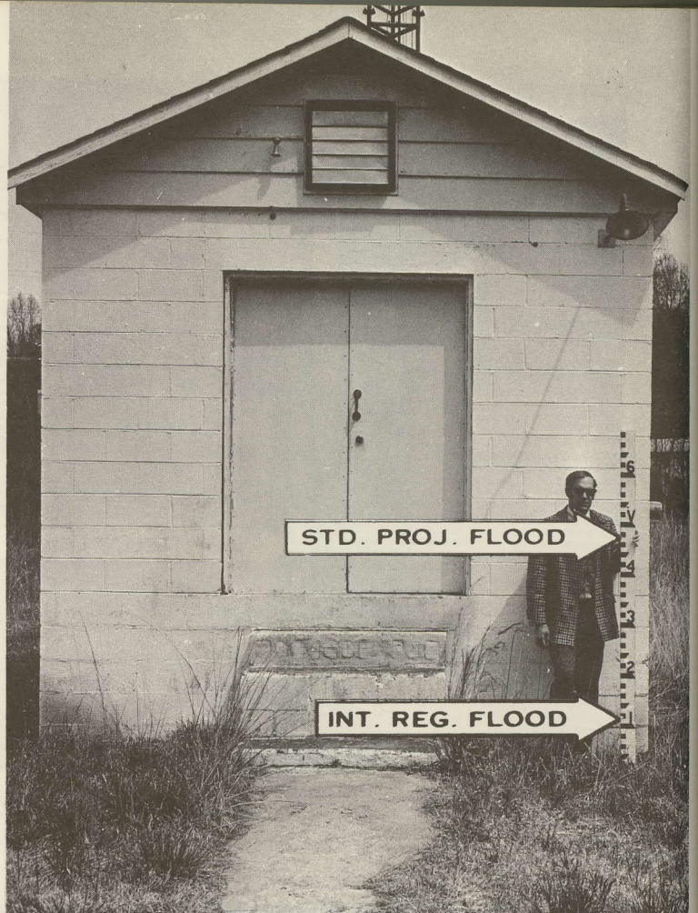
Radio Tower near intersection of Milbourne Road and Park Street (Va. Route 631)
